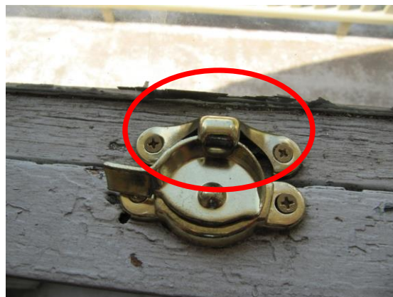
Shown locked; note lock "hood" over arc.
