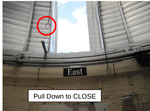
Dome Slit cover shown CLOSED, but NOT latched (on left)
