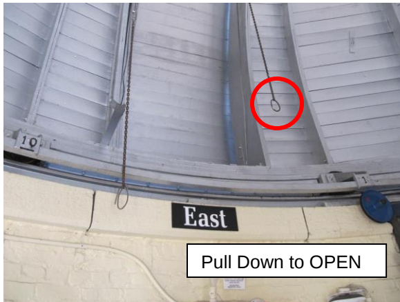
Dome Slit cover shown CLOSED, but NOT latched (on left)
